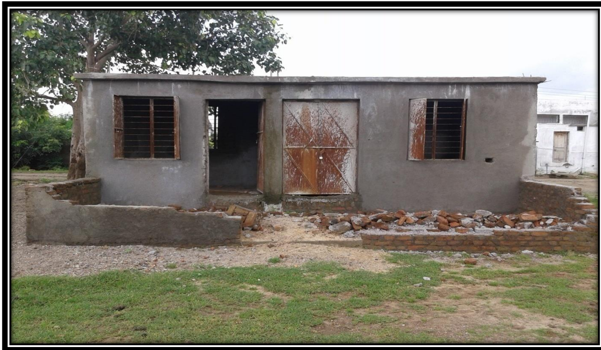
MDM: kitchen shed-cum-store under construction
