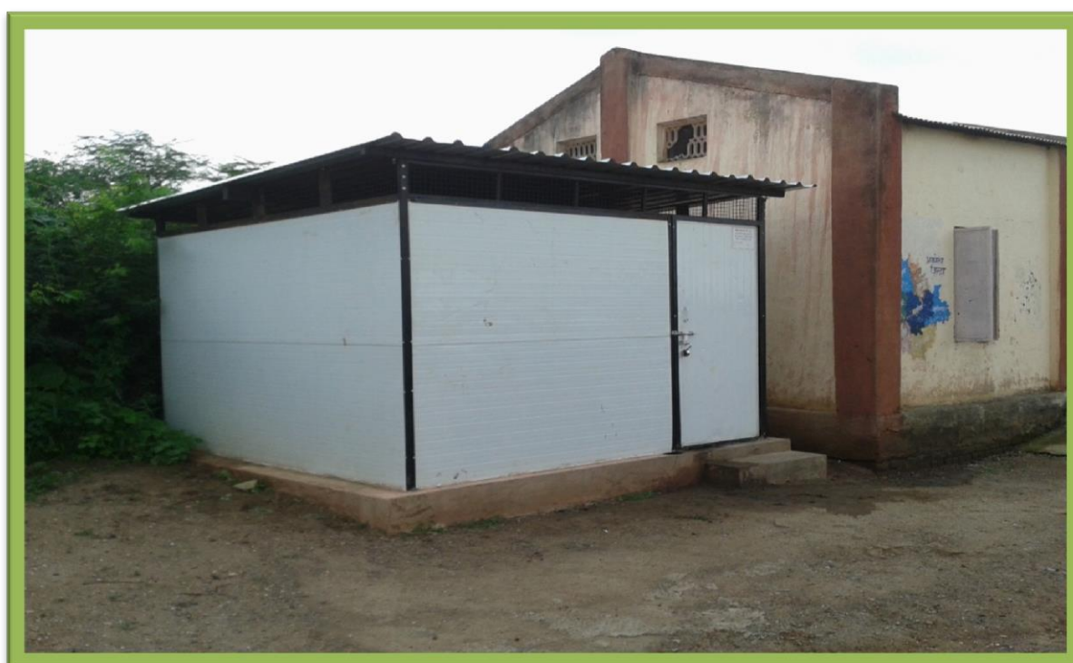
MDM: New type of fibre kitchen shed
