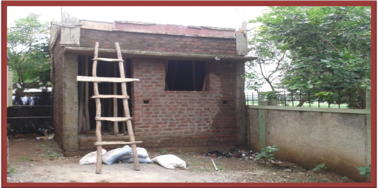
MDM: Kitchen Shed Under construction
